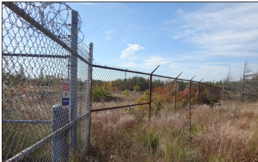
Training Area in the Western Portion of MCRC Brooklyn
