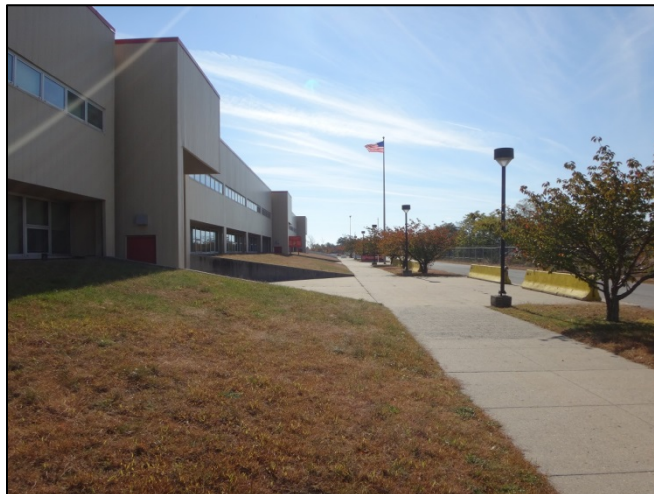
Administration Building Proposed for Exterior Renovation
